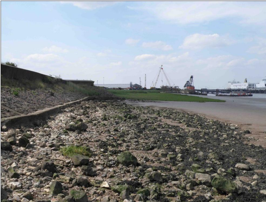
Photograph 2. Foreshore at North Killingholme, Humber Estuary showing exposure of the toe of the sea wall as a result of lowered mudflats. This mudflat lowering is attributed to 'coastal squeeze'.
