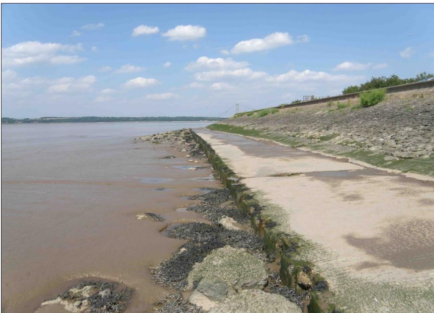
Photograph 3. Foreshore at Barton on Humber, Humber Estuary showing sea wall toe extension and further exposed toe. Again, this mudflat lowering is attributed to 'coastal squeeze'.
